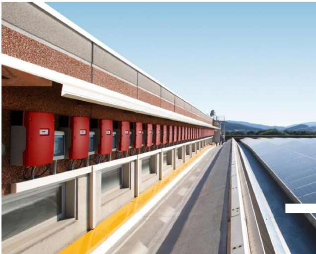
Mounted inverters close to PV modules
